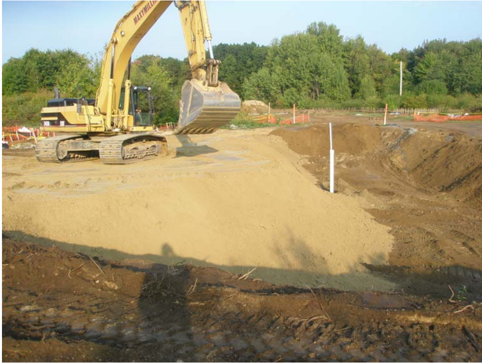
Photograph 3 –Backfilling Excavation
