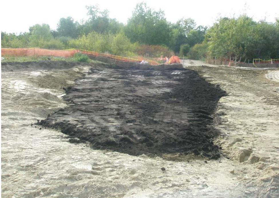
Photograph 4 – Completed Wetland Restoration Area
