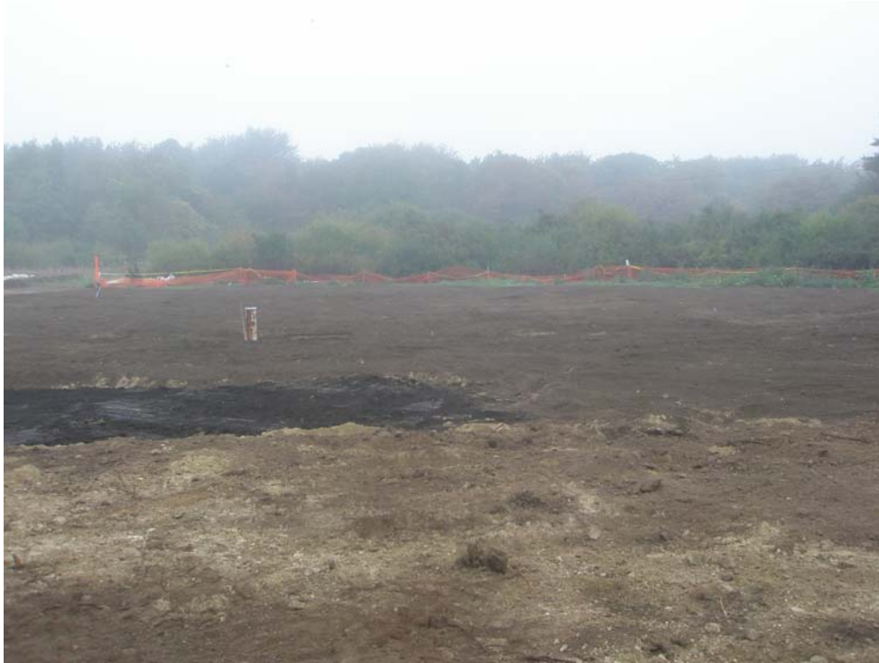
Photograph 5 – Finished Excavation Area Grades
