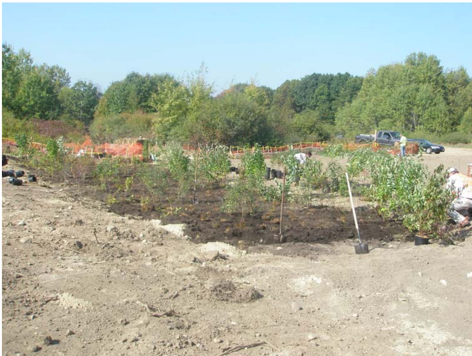
Photograph 6 – Completed Wetland Restoration
