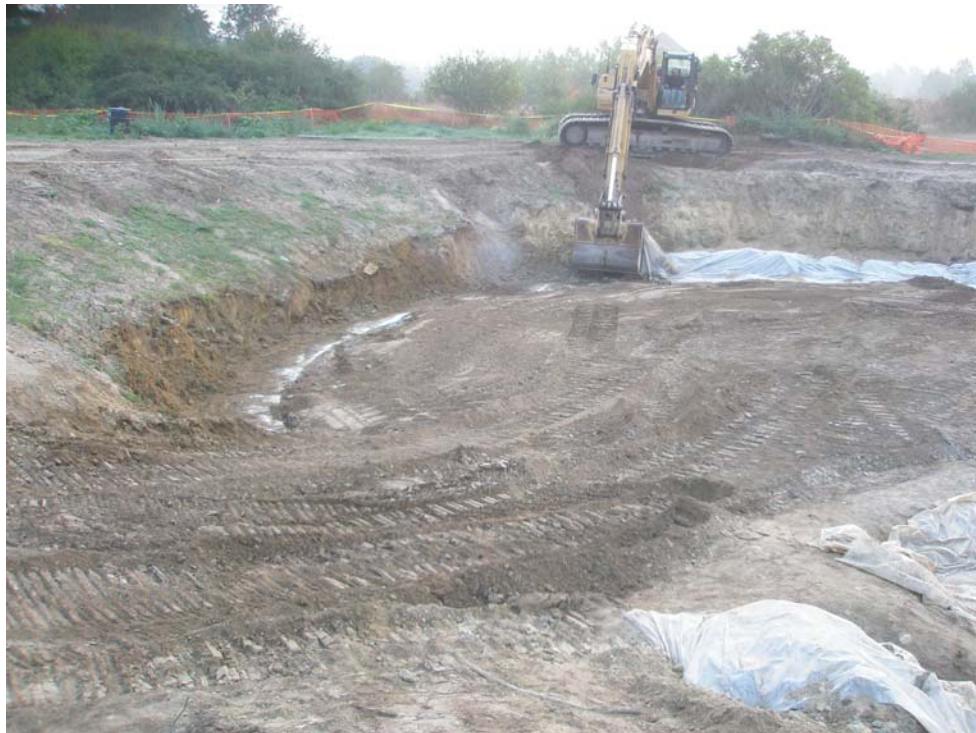
Photograph 2 – Removing Residual Soil for Disposal
