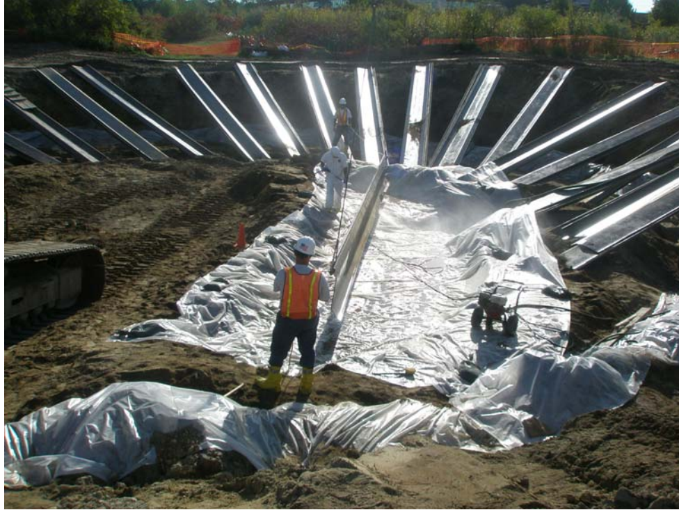
Photograph 1 –Sheet Pile Decontamination
